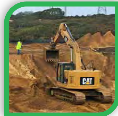
Construction of expanded percolation pond to accommodate waters from four existing and two future ASR wells.
